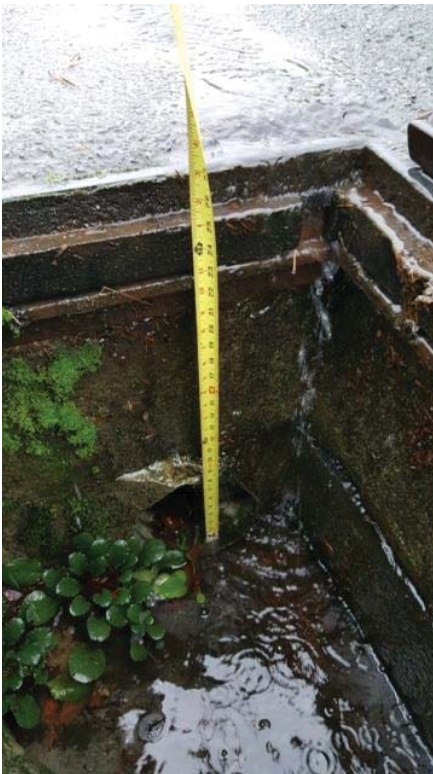
2 - Existing CB 8" CMP Outlet
