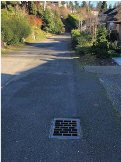
6 - Existing CB Downstream, Looking East.
